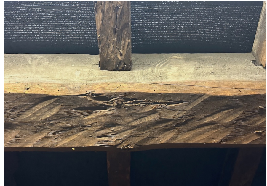
30. Detail of original roof timbers showing adze marks & modern felt.
