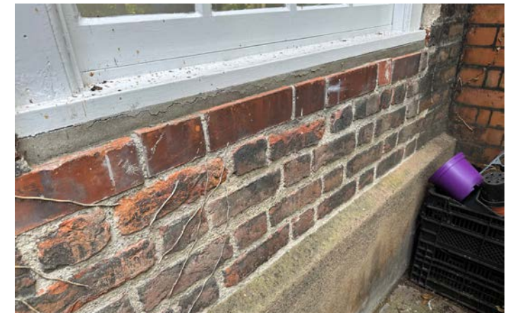
53. Detail of 2015 test repointing using lime mortar.
