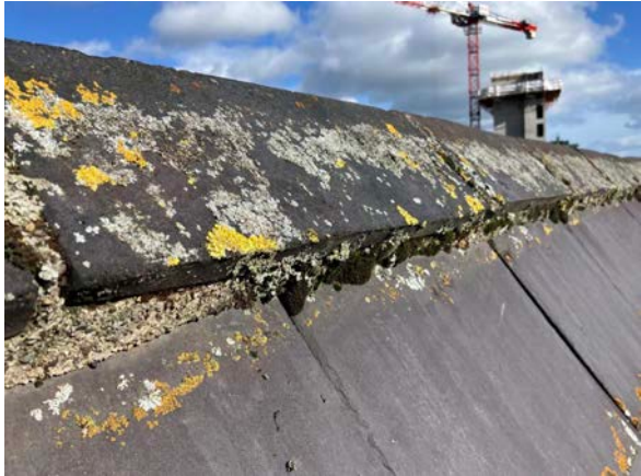
32. View along ridge showing pointing intact.
