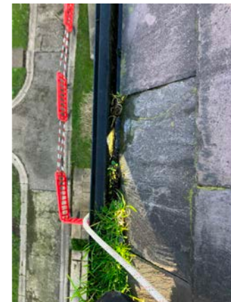
38. Detail of blocked gutter.
