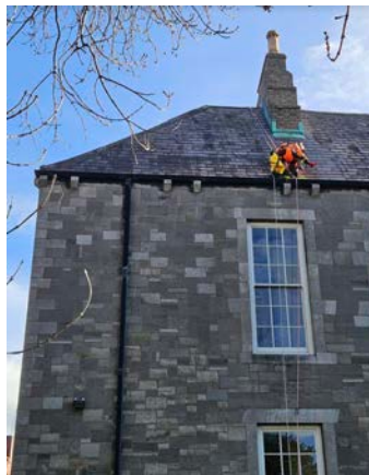
35-37. Niall McDonagh undertaking recent roof inspection, cleaning and repairs using safe rope access method where installation of scaffolding or hoist hire would be needed.
