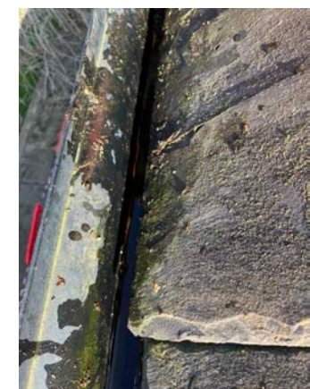
39. Gutter following cleaning.
