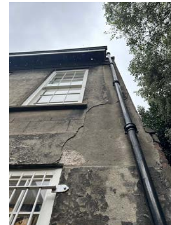
27 & 28. Views of cracked ruled ashlar render to east range.
