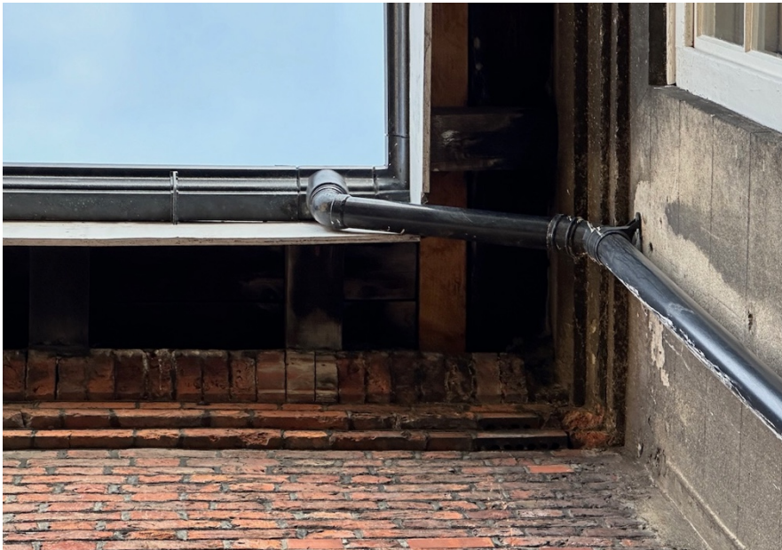
31. Detail of modern eaves board and guttering to garden facades.
