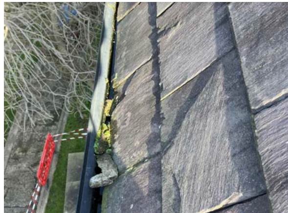
33. View of blocked gutter along west wall.
