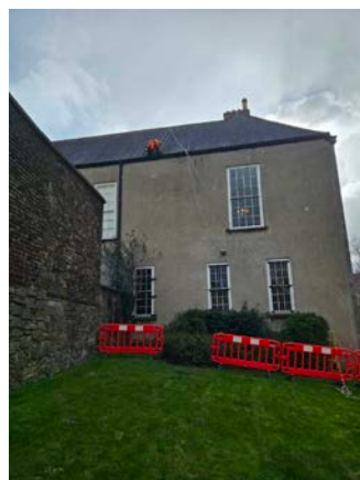
35-37. Niall McDonagh undertaking recent roof inspection, cleaning and repairs using safe rope access method where installation of scaffolding or hoist hire would be needed.
