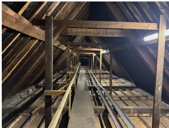
42. View along north range attic with queen post.
