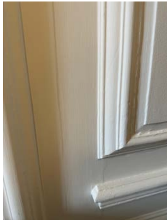
76. Detail of bolection moulding to architrave.
