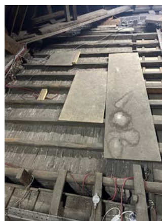
46. Evidence of drip in south range.
