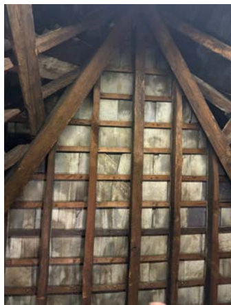
44. Unfelted slating to south range.
