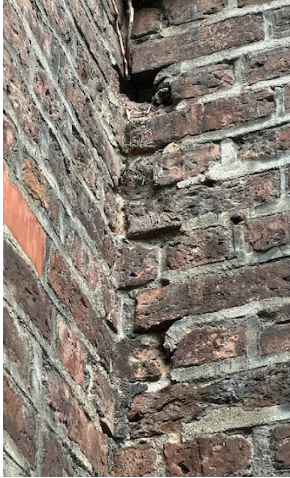
49 & 50. Views of hard cement pointing and missing joints and bricks to corners.
