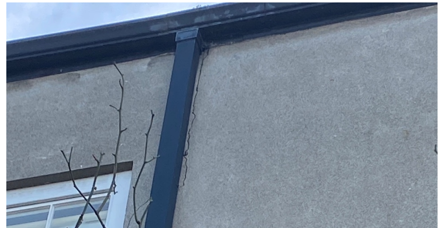
40. Detail showing cracked render under downpipe to north wall.
