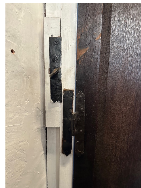
87. Wrought iron hinges to shutters.
