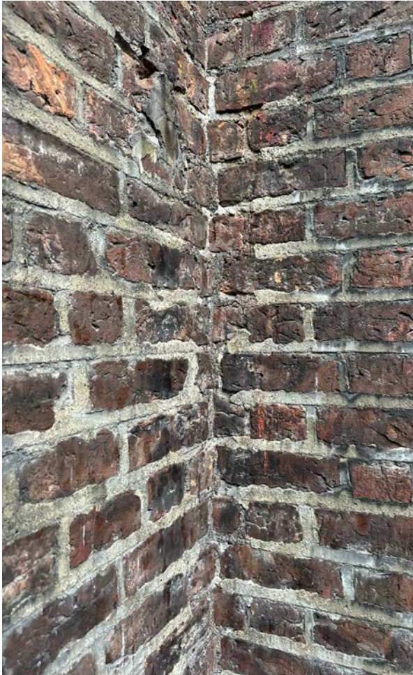
49 & 50. Views of hard cement pointing and missing joints and bricks to corners.
