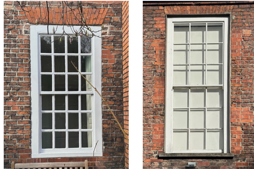
54 & 55. Early 18c. (left) and 19c. (right) replacement sash windows.
