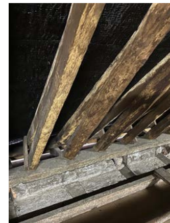
47. Unwrought timber without birdsmouth detail in roofspace.
