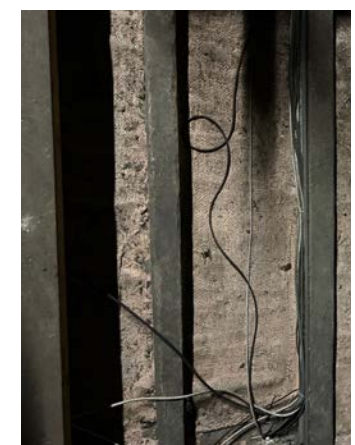
48. Gypsum treated hessian over reading room for fire proofing.
