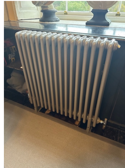
99 & 100. New electric heater and installation in Old Reading Room.
