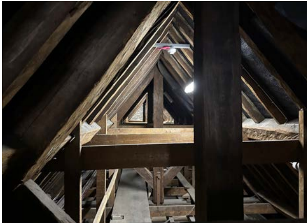
41. View along west range attic with king post trusses.
