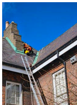
35-37. Niall McDonagh undertaking recent roof inspection, cleaning and repairs using safe rope access method where installation of scaffolding or hoist hire would be needed.
