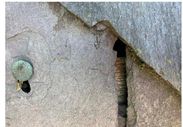
34. Detail of slipped slate showing gap for water ingress.
