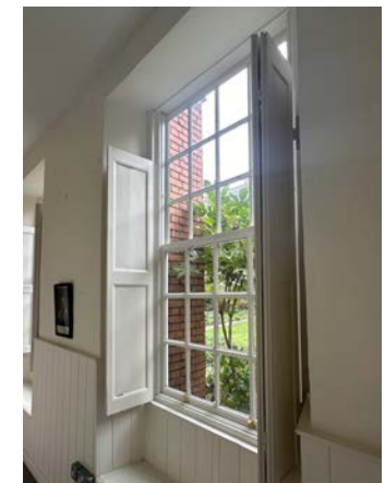
80. Detail of repaired sash window to garden corridor.
